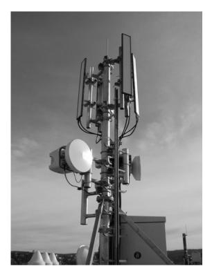
Figure 13-4: A Base Station Sector Antenna Array (Courtesy of European Antennas Ltd.)
